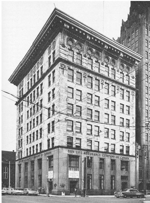
(Left) Circa 1950s view of the Sun Life Building, showing the enormous sheet-copper cornice and terra-cotta brackets still intact. (Toronto Region Architectural Conservancy, Terra Cotta – Artful Deceivers, p. 63).
